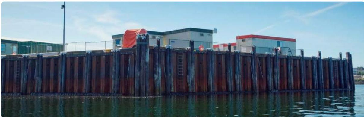
Photo 4. Completed Phase 1A Sheetpile Perimeter Wall around South Jetty
